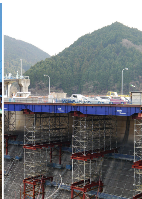
Dom flood control construction/Hi-RoRo method®
